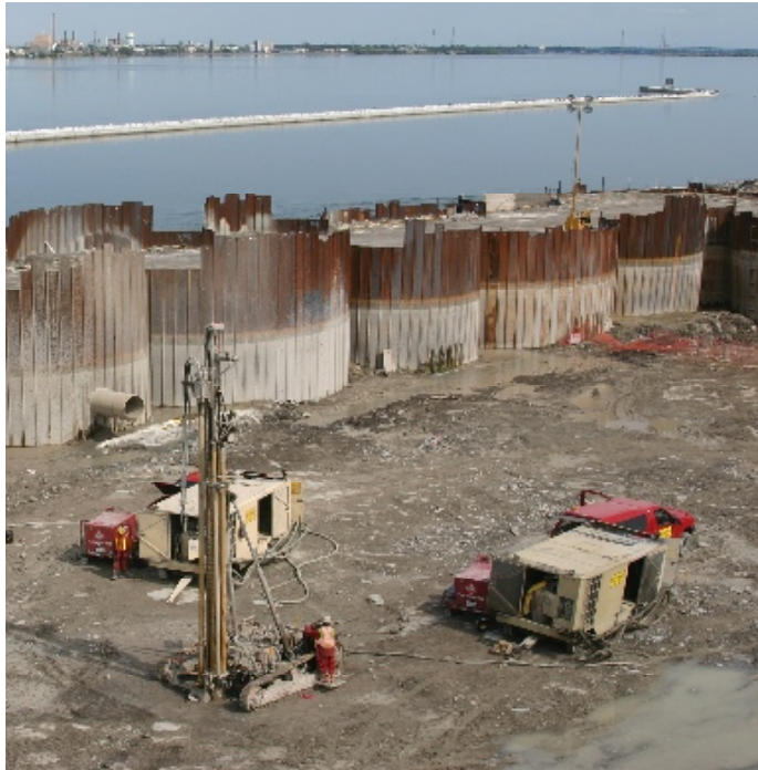
The completed cofferdam, drained of water.
