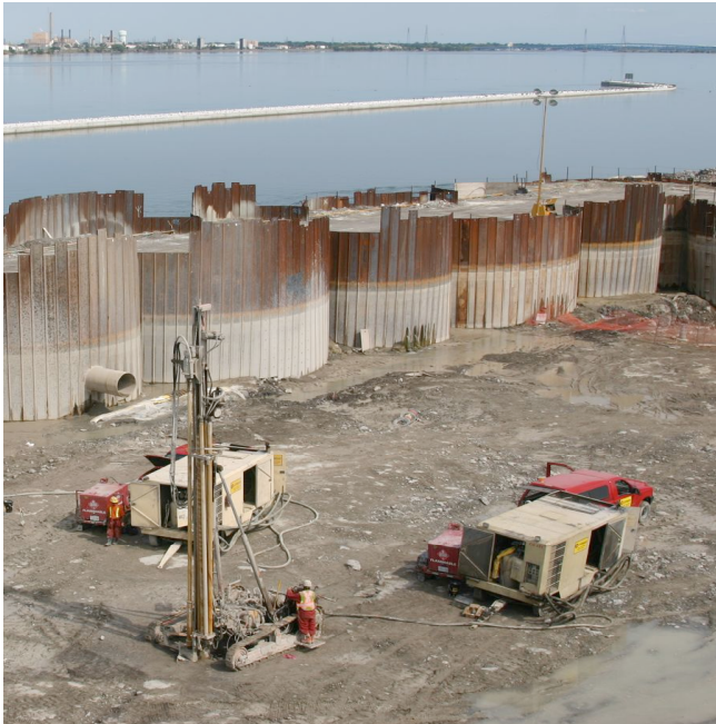
The completed cofferdam, drained of water.
