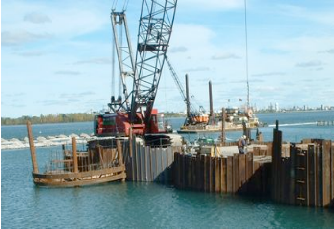
The cofferdam during construction.
