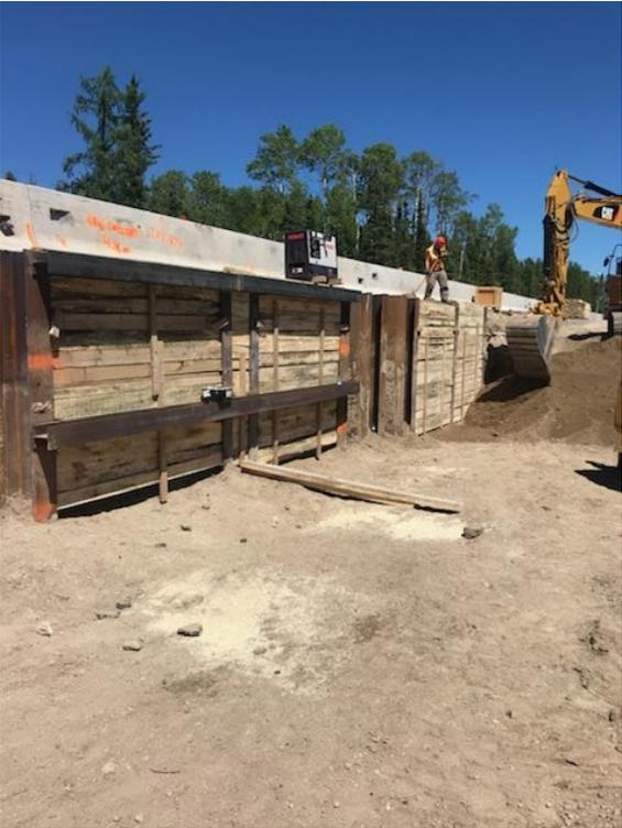
Figure 10: Shoring System Approximate 10-FT Excavation Depth
