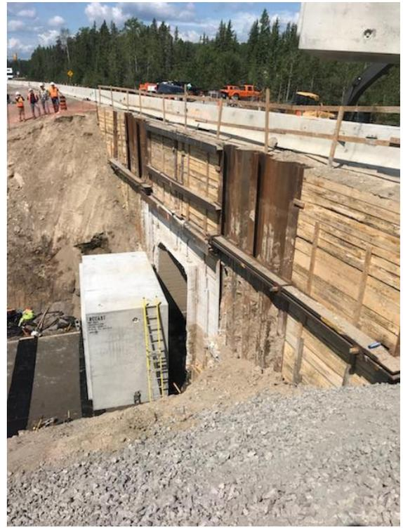
*Figure 11: Completed Shoring Wall at HWY 11 Culvert 119*
