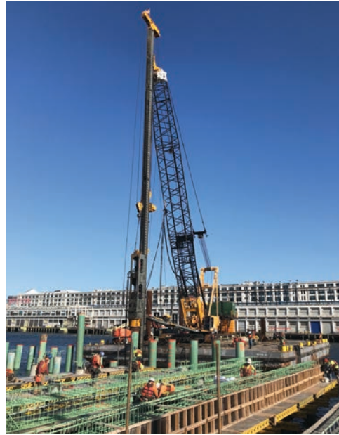
A Coastal Marine rig impacting piles
