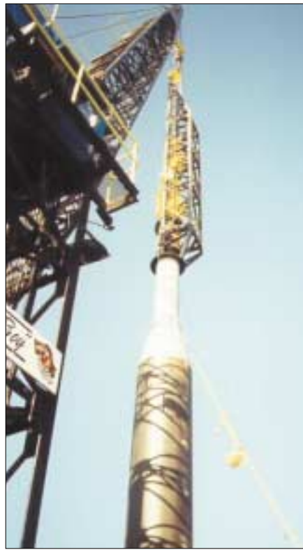
B-6505 Preparing to drive a 72" diameter Pile 100 ft into Chesapeake Bay
