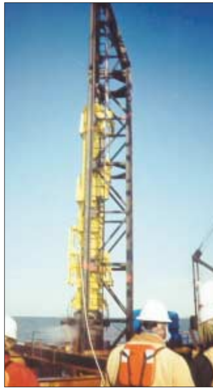
The B-6505 after driving the 72" Pile to 100 ft penetration
