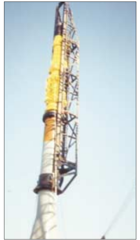
Driving the Pile with a Berminghammer B-6505 Smokeless Hammer
