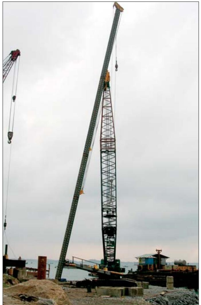
*The L23 lead system, drilling six piles a day on a project in Vietnam. One of the obstacles to overcome was the distance from the crane that drilling had to take place. Bermingham designed and fabricated a 7.6m (25ft) three-stage spotter so the client could work at more than a 15m (50ft) radius from the center of the crane.*
