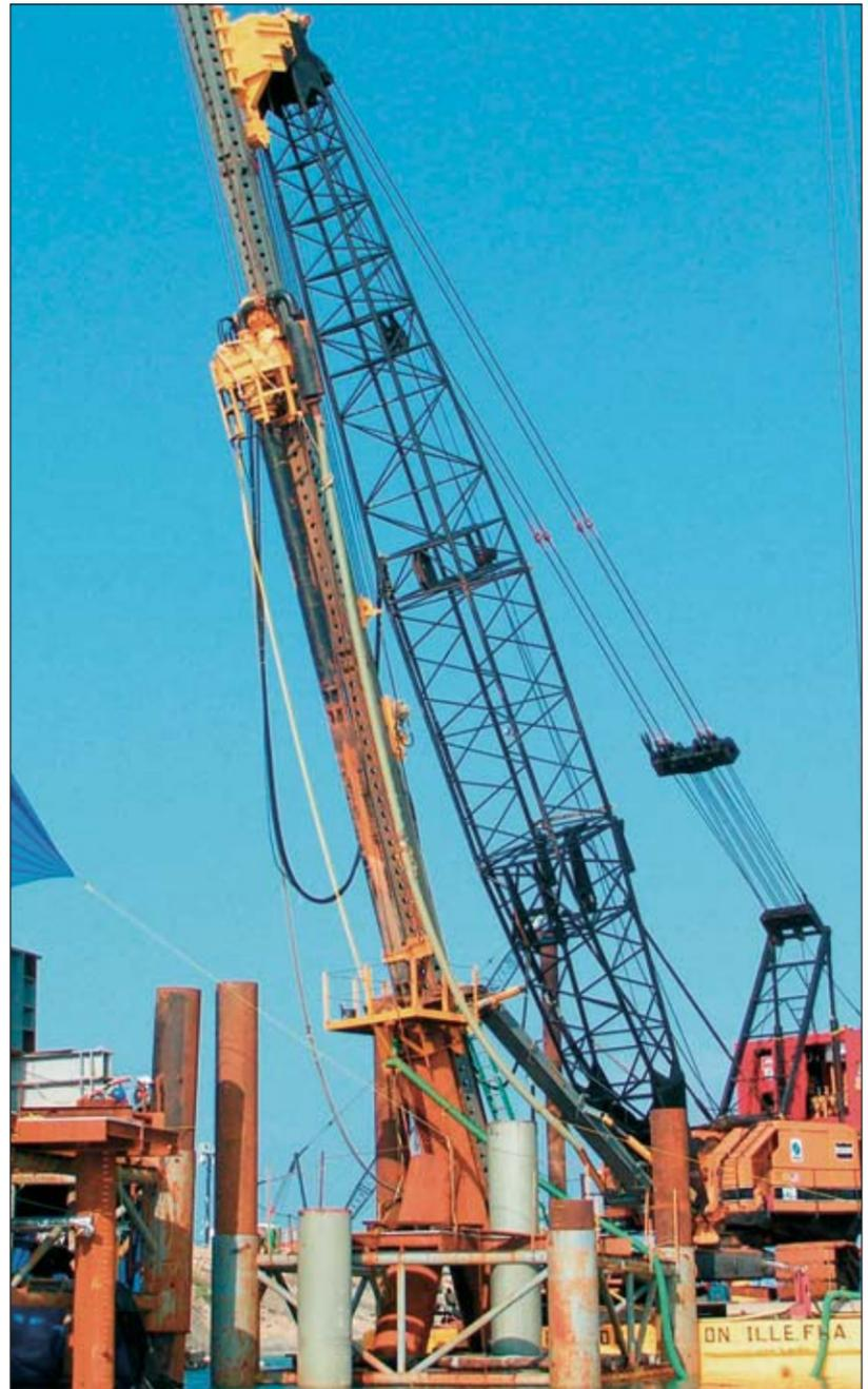
The Berminghammer 60/60 drilled rock sockets to a depth of 46m (151ft).
