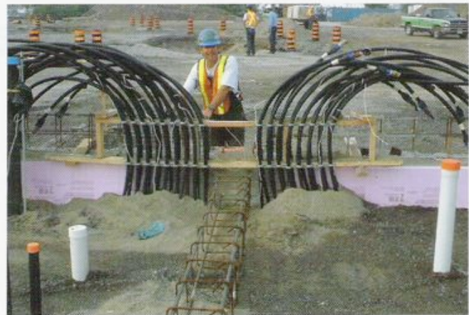
Preparing to Hook-Up Polyethylene Pipes from Piles to Manifold
