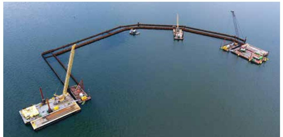
Top: Falsework to guide the sheet piles into place had to be installed on a barge between the inner and outer walls. Above: An overhead view of the structure nearing the halfway point in construction.
