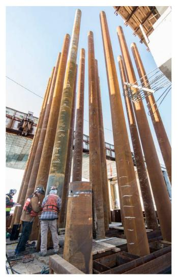
capacity for the specified tip elevation. To surmount this, the owner added more piles, and JT Cleary once again re-designed the cofferdam, and the project proceeded smoothly and without issue.
