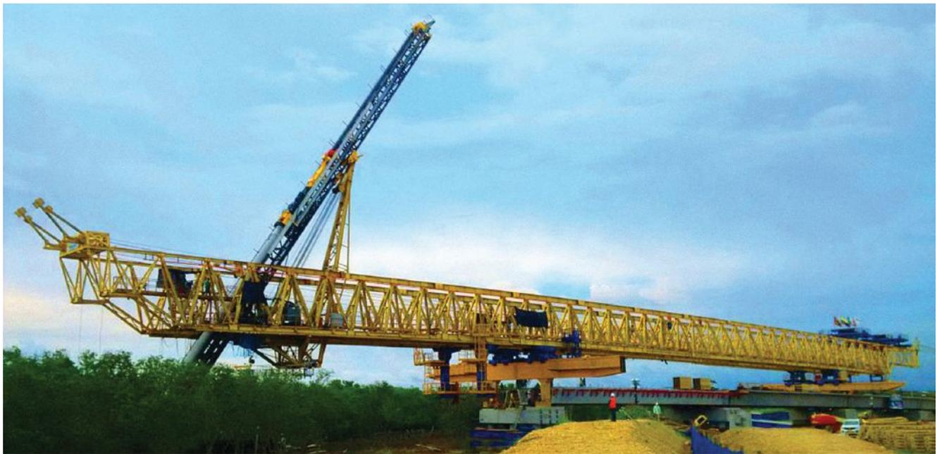
**In** 2015, Stefano Gabaldo of Birmingham was contacted by DEAL (of Italy) to assist with the piling portion of a new Beam Launcher project in Cartegena, Colombia. DEAL parent company of Rizzani de Eccher was to build a 5 km bridge with bents spaced at 37 meter increments. This bridge was the final section of the highway connecting Barranquilla to Cartagena to be upgraded.
