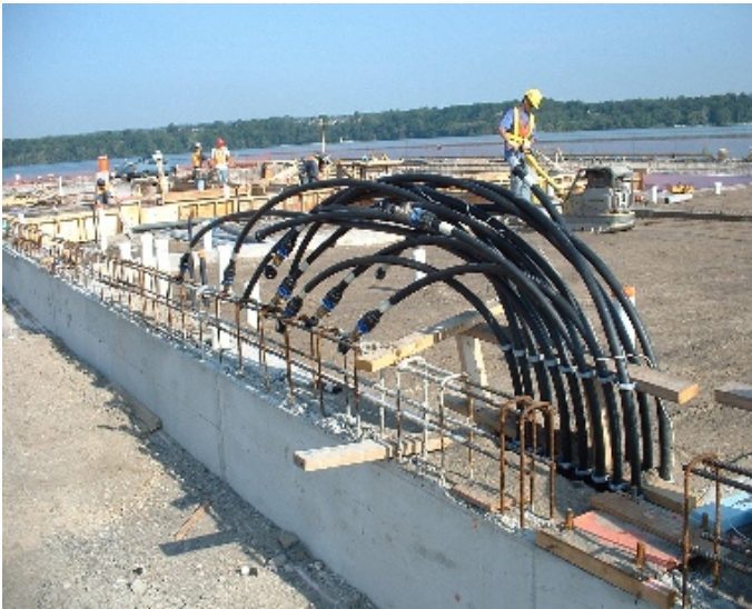
Geo-exchange circuits (left) exit the piles and lead to the manifold (right).
