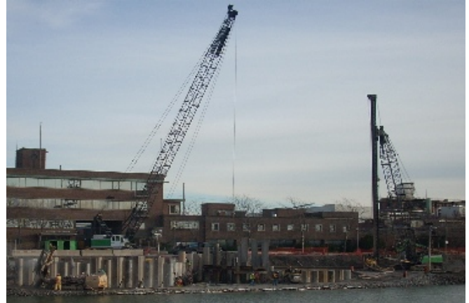
The combi wall during construction.
