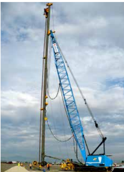
L-23 VTL for Wick Drains
