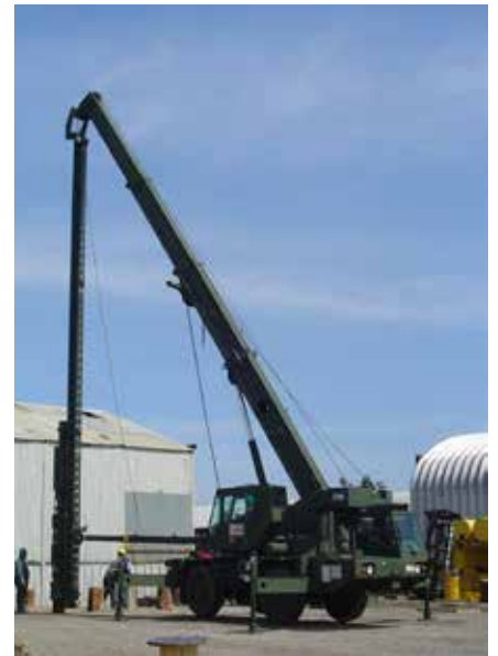
C-12M Fixed for Piling
