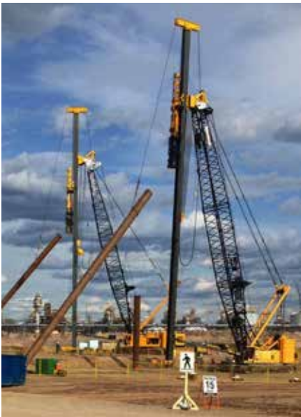
L-27 VTL for Piling 36"
