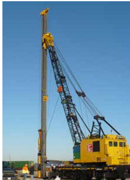
L-18 VTL for Railroad Piling
