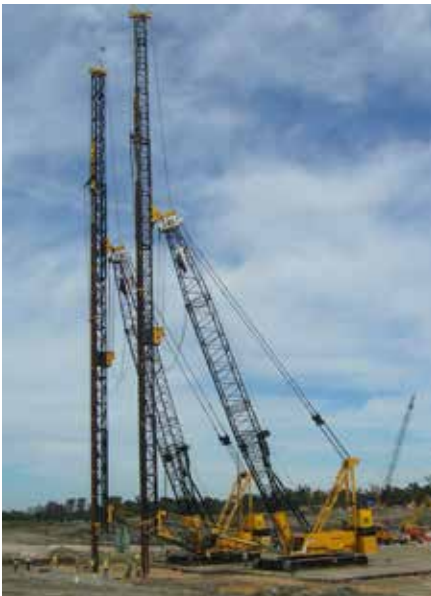
VTL for Piling
