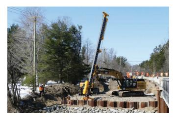
It's the latest offering in the company's line of excavator mounted leads (EML) and was a perfect fit for the Cat 349 hydraulic excavator Polaris already had on hand.
