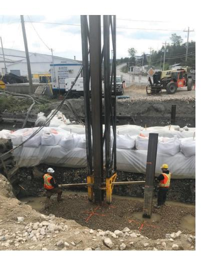
"The B21 is 72 kilojoules [kJ] and the government had a maximum rated pile hammer energy of 84 kilojoules," said Tripp. "We were driving a 12-inch 74-pound-foot H-pile and we couldn't exceed that rating. The next size hammer, the B32, had 110 kJ."
