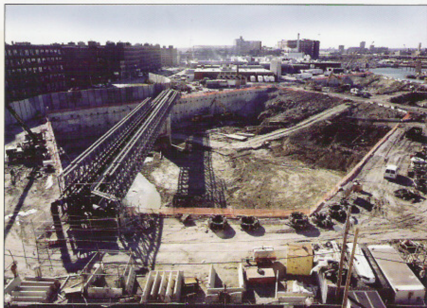
Partially excavated Casting Basin looking west toward the Fort Point Channel.
