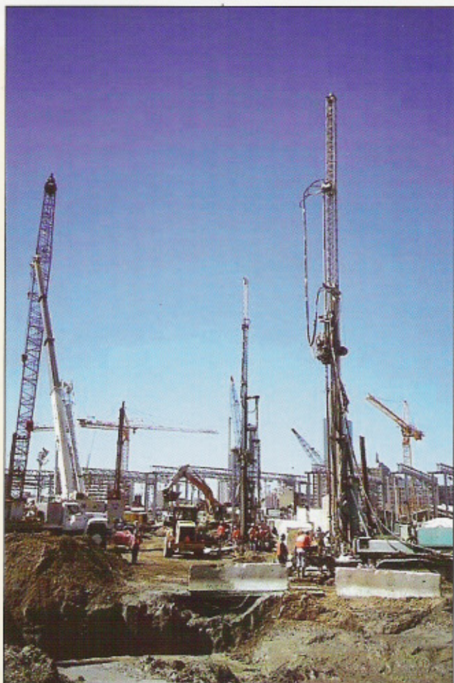
Nicholson's jet grouting activities at C09A7 project.
