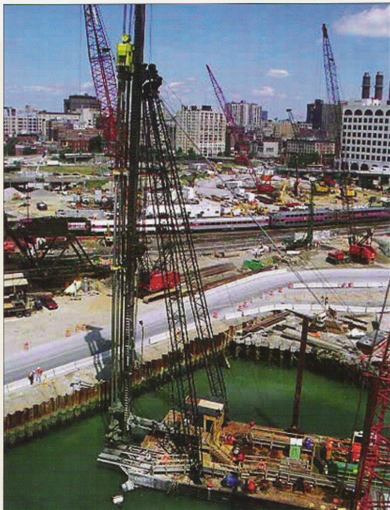
Barge-mounted soil-mixing rig working at the Fort Point Channel.
